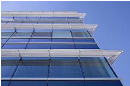
Exterior Light Shelves - Green Office Building, Denver, Colorado
