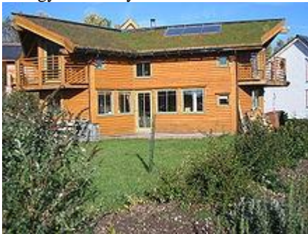
An eco-house at Findhorn Ecovillage with a turf roof and solar panels
